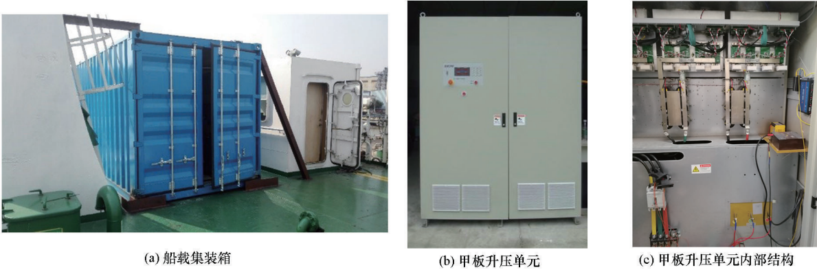
图 9 甲板升压单元实物 Fig.9 Physical picture of deck booster unit
