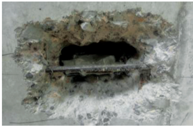
图 9 管道灌浆不密实钻孔验证 Fig.9 Verification of uncompacted pipeline grouting
